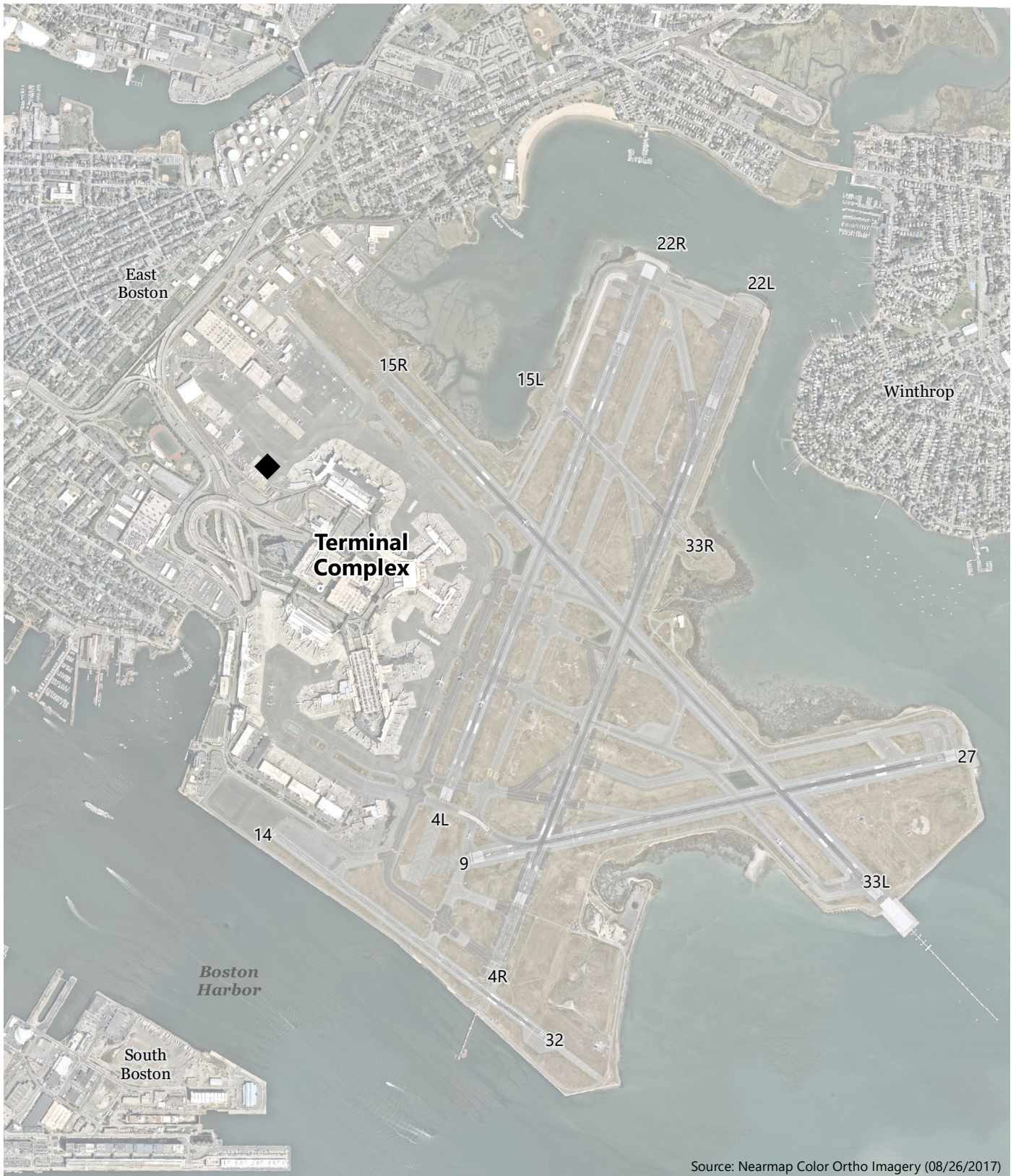
FIGURE 9-6 Terminal E Modernization Project
