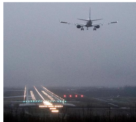
CAT III Instrument Landing System. Source: Massport.
