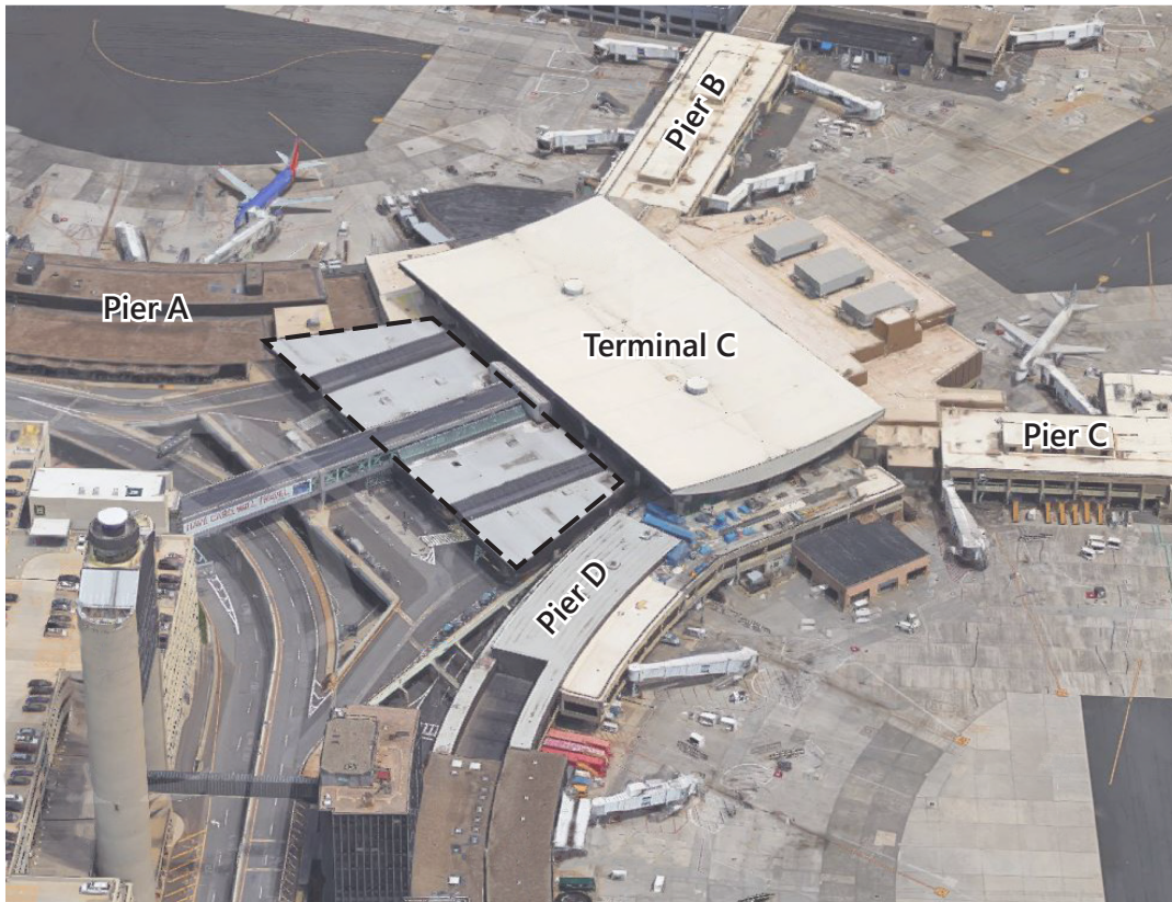
Existing Terminal C
