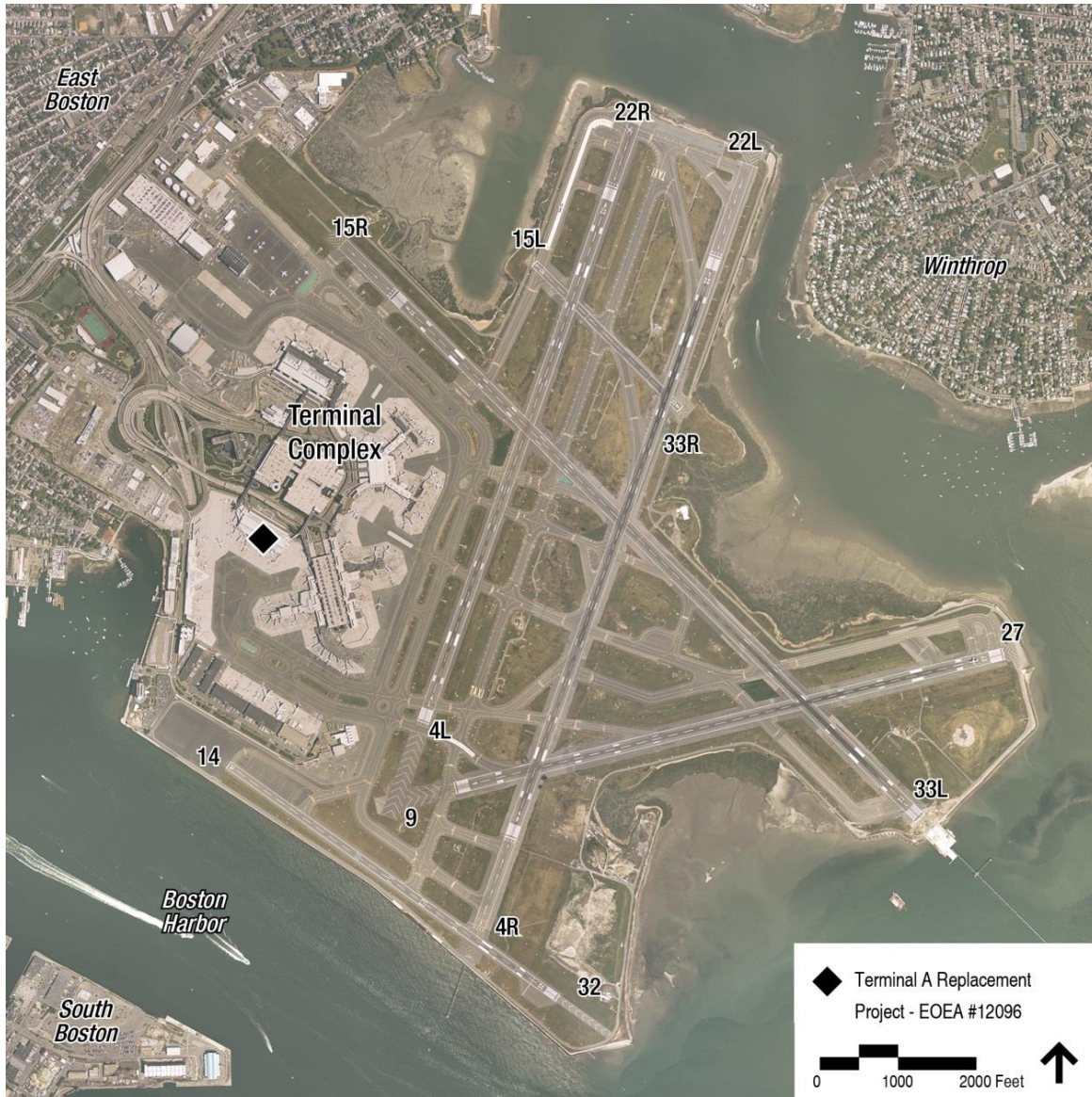
Figure 9-3 Replacement Terminal A Project
