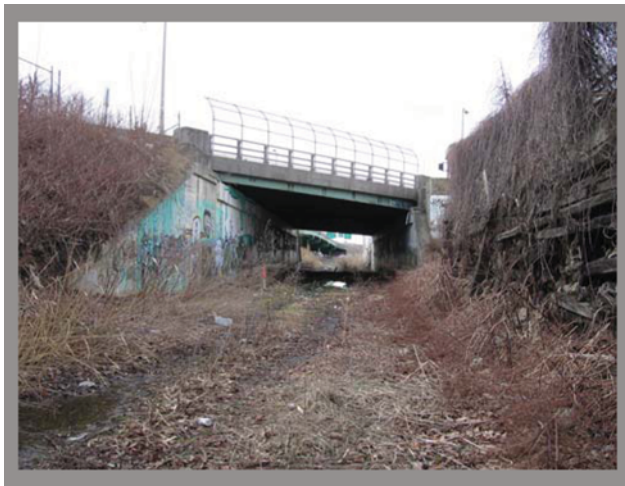
View of Bridge Looking South Bennington Street/Neptune Road
