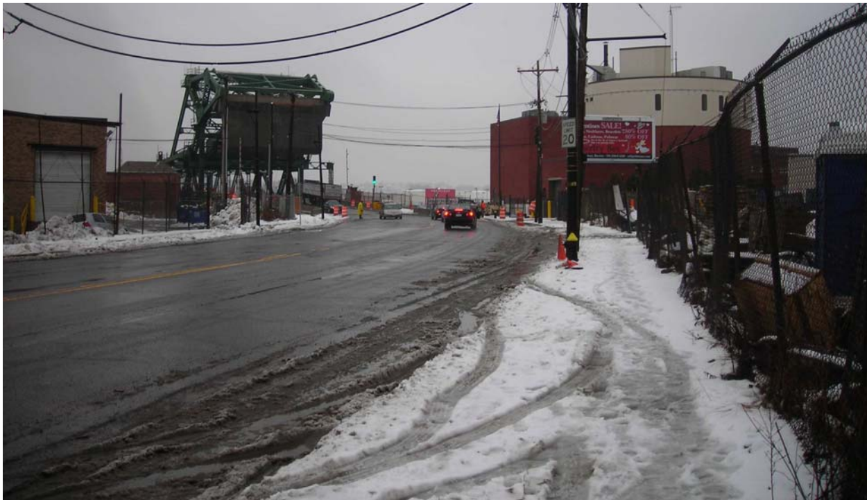
Chelsea Street northbound near Location 1 (approaching Chelsea Street Bridge)
