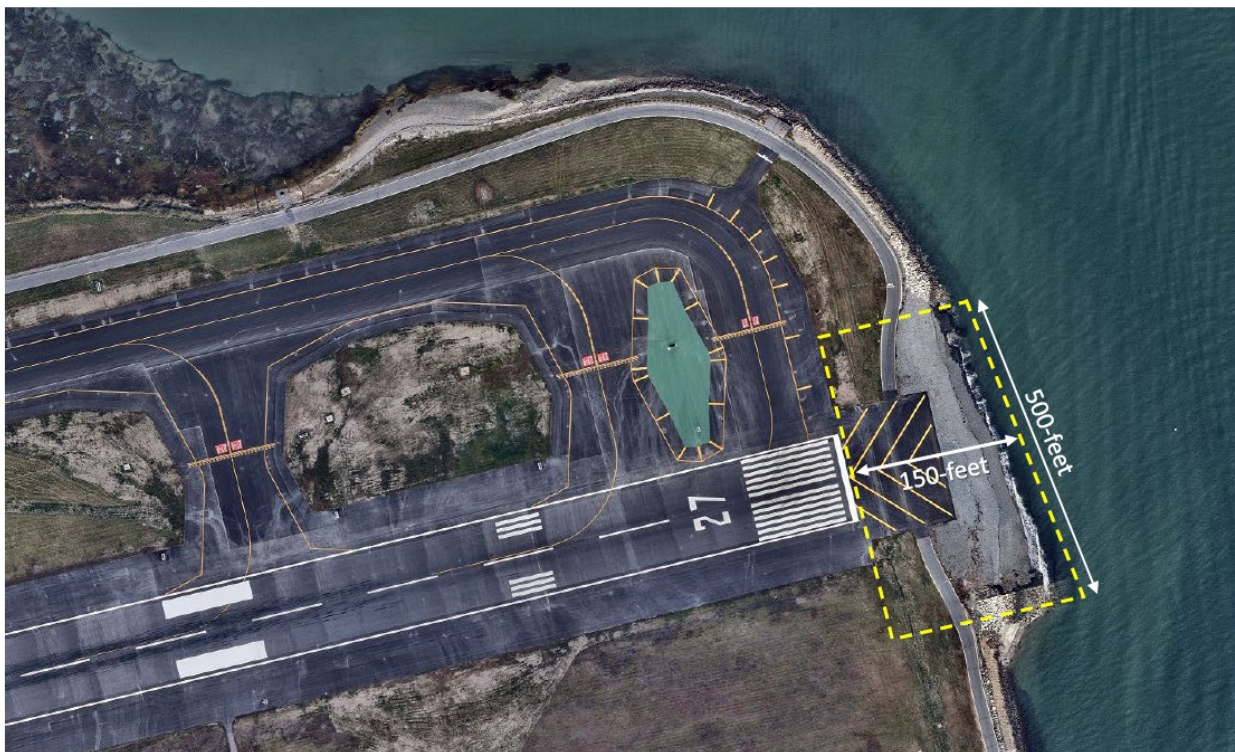
Figure 2-1 Runway 27 End - Existing Runway Safety Area
