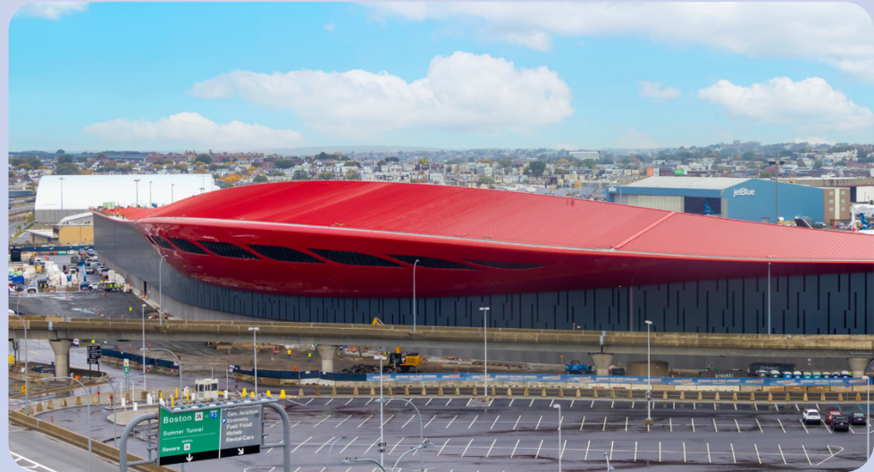
View of the Terminal E Modernization project
