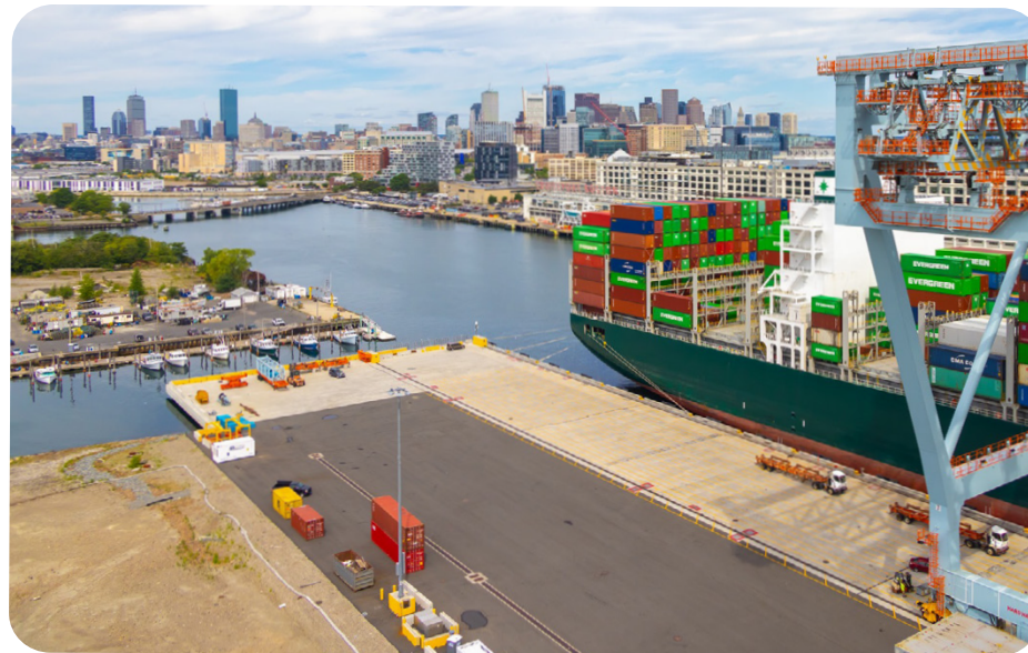
Conley Terminal's new Berth 10
