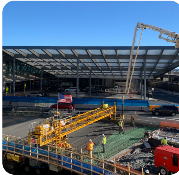
Construction of the Terminal B-to-C Roadways Improvement project
