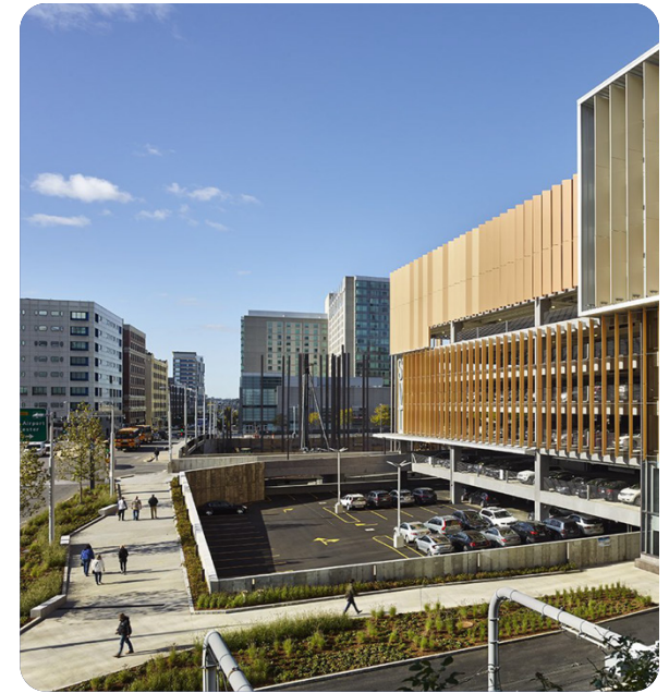
Parcel D-4 site for a future mixed-income housing development
