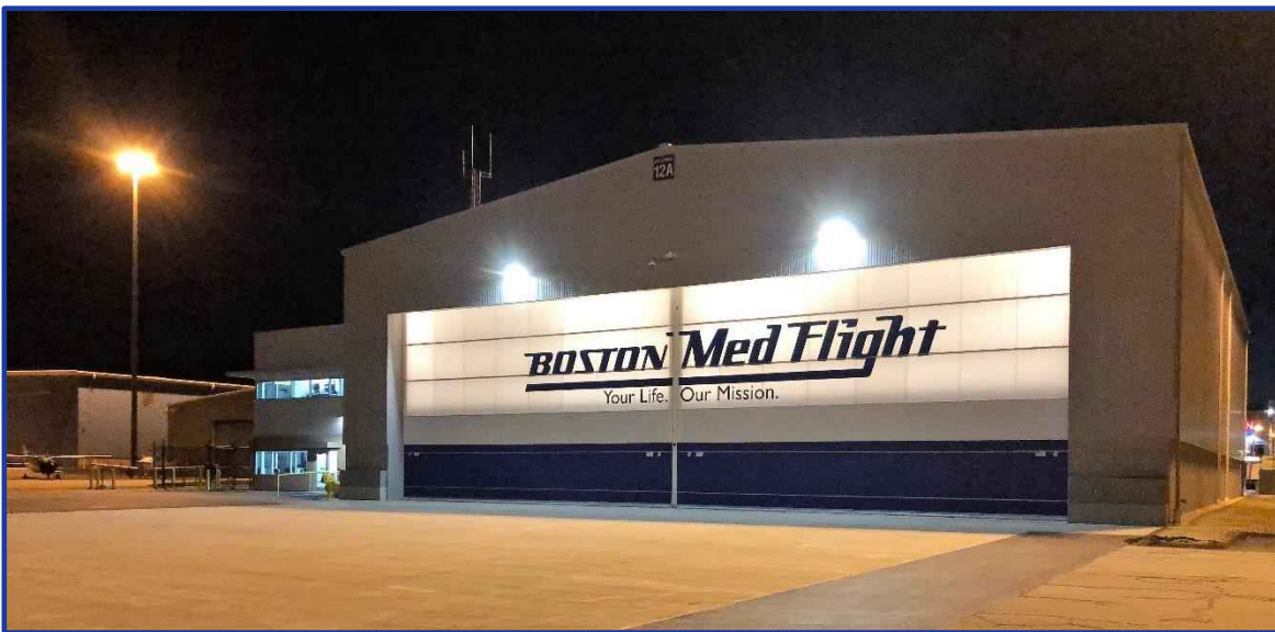
Figure 11-9 Translucent Hangar Door Allows Natural Light to Enter Boston MedFlight's Hangar
