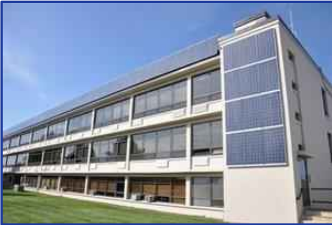
Figure 11-7 Solar PV Panels on Hanscom Field Civil Air Terminal
