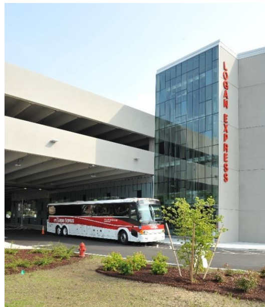
New Framingham Logan Express 1,100-space garage. Source: Massport
