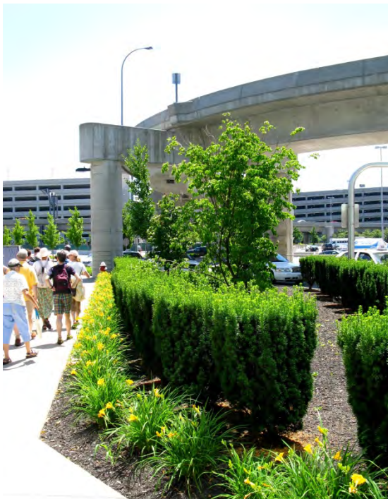
Pedestrian walkway from Terminal C to Terminal E, 2010.
